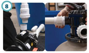
Using PVC primer and glue, install assembly #4 to the outlet on the pump. Thread the union on assembly #4 to the fitting on the pump port of the filter. **DO NOT OVERTIGHTEN!**
