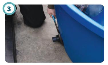
Tighten the bulkhead nut from the outside of the tank, hold the body of the bulkhead assembly securly from inside the tank. DO NOT OVERTIGHTEN!
