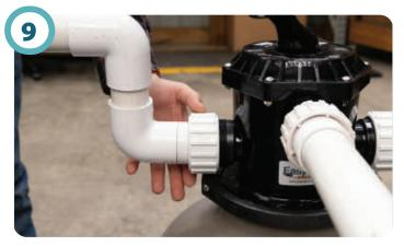
Connect assembly #1 to the return port on the filter. **DO NOT OVERTIGHTEN!**
