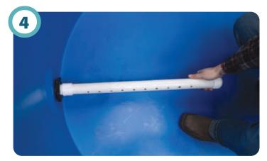
Inside of the tank, install assembly #2 into the bulkhead assembly. Adjust it so the holes are facing into the planned current or rotation of the water. Do not point straight up or straight down.
