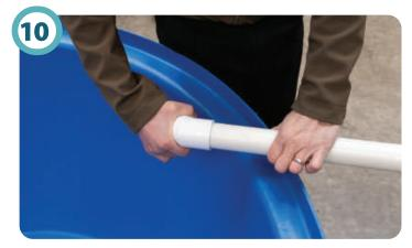
Slide the 45 degree elbow on the end of assembly #1. **DO NOT GLUE.** Orientate the elbow to promote the direction of current/rotation in the tank that is desired.
