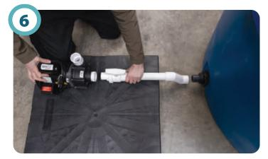
Place assembly #3 between the tank and pump inlet Using PVC primer and glue, install assembly #3 to the bulkhead assembly on the tank and into the inlet on the pump.
